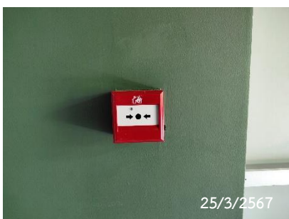
Fire Alarm Manual Station
